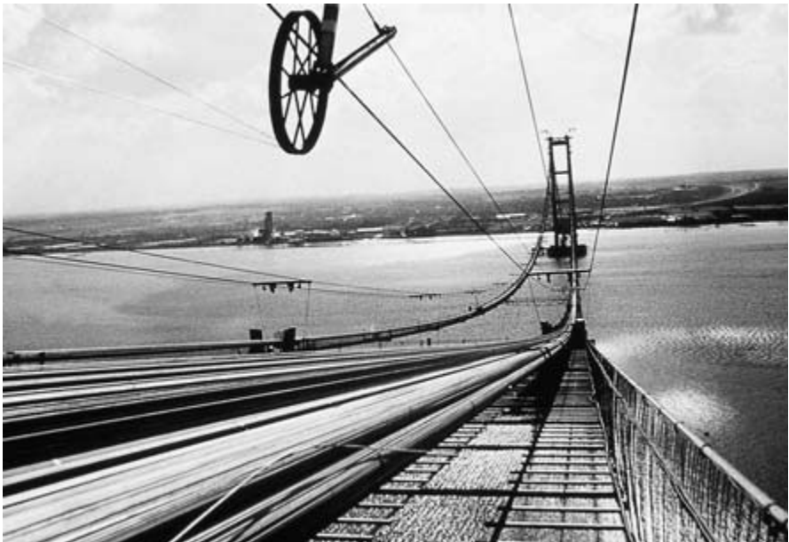
Figure 1.23 Cable Spinning for Humber Bridge.
