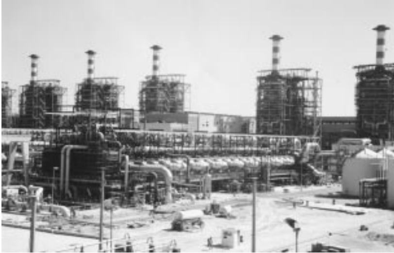
FIGURE 20.6.2 One of the six units of the 346,000 m 3 /day MSF desalination plant Al Taweelah B in Abu Dhabi, United Arab Emirates. (Courtesy of Italmimpianti S. p. A.) It is a dual-purpose plant, composed of six identical power and desalination units. Five of the six boilers are seen in the background. The desalination units were in 1996 the largest in the world. They have 17 recovery and 3 reject stages and a performance ratio (PR) of 8.1. The plant also produces 732 MWe of power.
