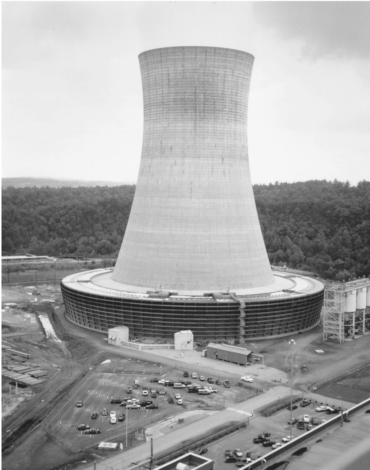
FIGURE 4.8.8 A natural-draft cross-flow cooling tower for a power plant.
