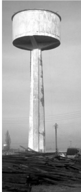
Figure 1.1.2 This reinforced-concrete tank on a 40-ft-tall single concrete column, located near the Valdivia Airport, was undamaged by the Chilean earthquakes of May 1960. When the tank is full of water, the structure can be analyzed as a single-degree-of freedom system. (From the Steinbrugge Collection, National Information Service for Earthquake Engineering, University of California, Berkeley.)
