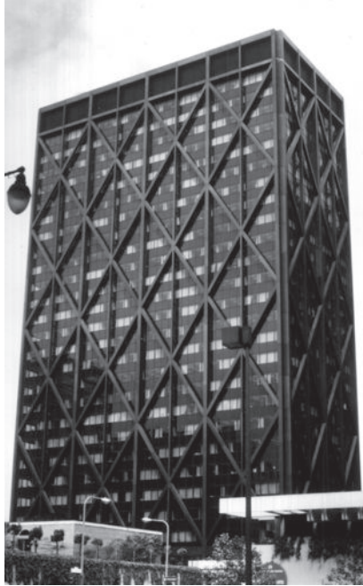
Figure 2.1.2a Alcoa Building, San Francisco, California. The fundamental natural vibration periods of this 26-story steel building are 1.67 sec for north–south (longitudinal) vibration, 2.21 sec for east–west (transverse) vibration, and 1.12 sec for torsional vibration about a vertical axis. These vibration properties were determined by forced vibration tests. (Courtesy of International Structural Slides.)
