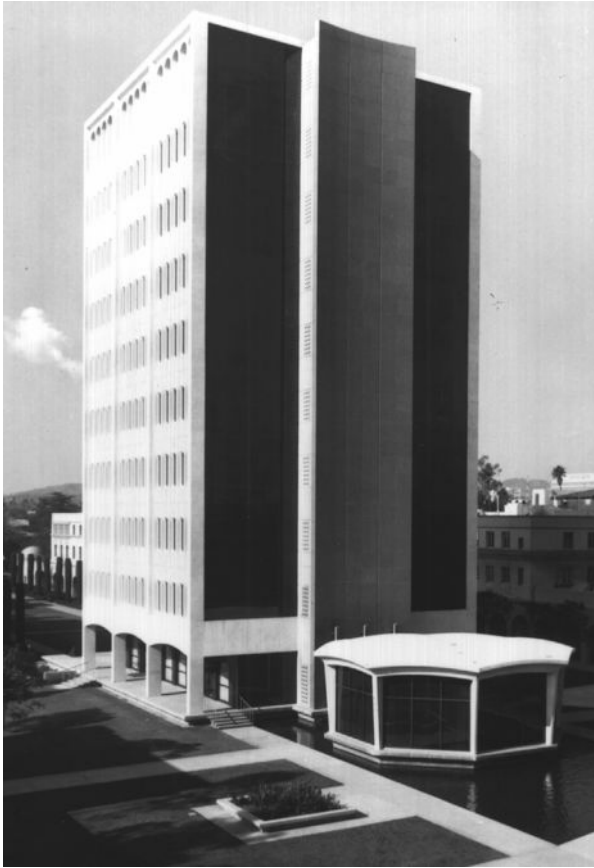
Figure 11.1.1 Millikan Library, California Institute of Technology, Pasadena, California. (Courtesy of K. V. Steinbrugge Collection, Earthquake Engineering Research Center, University of California at Berkeley.)
