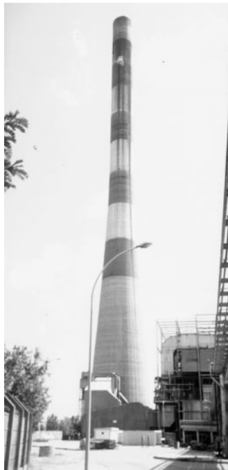
Figure 2.1.2f Reinforced-concrete chimney, located in Aramon, France. The fundamental natural vibration period of this 250-m-high chimney is 3.57 sec; it was determined from records of wind-induced vibration.
