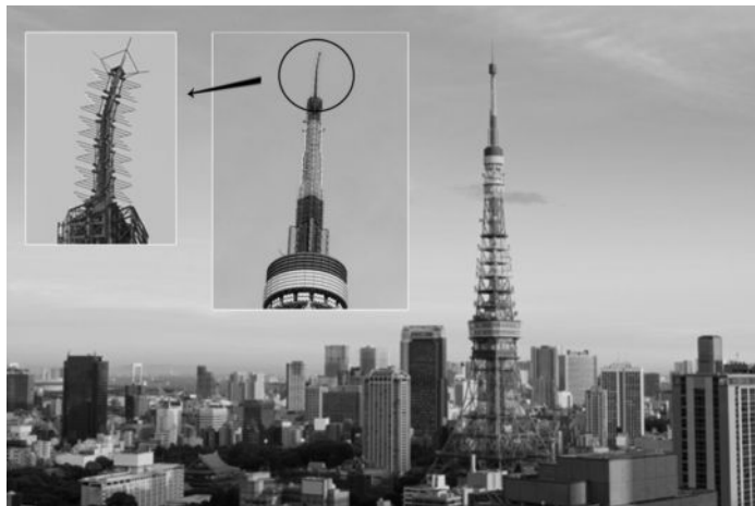
Figure 13.2.13 The 1091 ft-high Tokyo Tower performed well during the Tohoku, Japan, earthquake, March 11, 2011, Magnitude 9.0, except that the top part bent permanently. Shown is the tower before and after, with a second focus on the bend near the top. (Courtesy of C. D. James and C. Bodnar-Anderson, National Information Service for Earthquake Engineering, University of California, Berkeley.)
