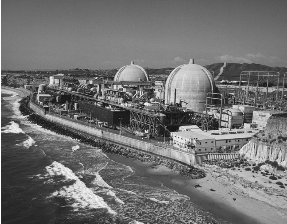
Figure 1.10.1 These two reinforced-concrete dome-shaped containment structures house the nuclear reactors of the San Onofre power plant in California. For design purposes, their fundamental natural vibration period was computed to be 0.15 sec assuming the base as fixed, and 0.50 sec considering soil flexibility. This large difference in the period indicates the important effect of soil–structure interaction for these structures. (Courtesy of Southern California Edison.)
