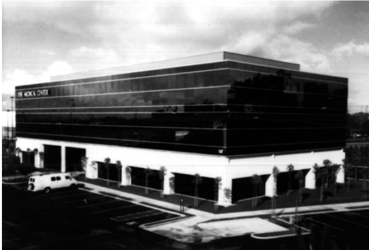
Figure 2.1.2c Medical Center Building, Richmond, California. The fundamental natural vibration periods of this three-story steel frame building are 0.63 sec for vibration in the long direction, 0.74 sec in the short direction, and 0.46 sec for torsional vibration about a vertical axis. These vibration properties were determined from motions of the building recorded during the 1989 Loma Prieta earthquake. (Courtesy of California Strong Motion Instrumentation Program.)
