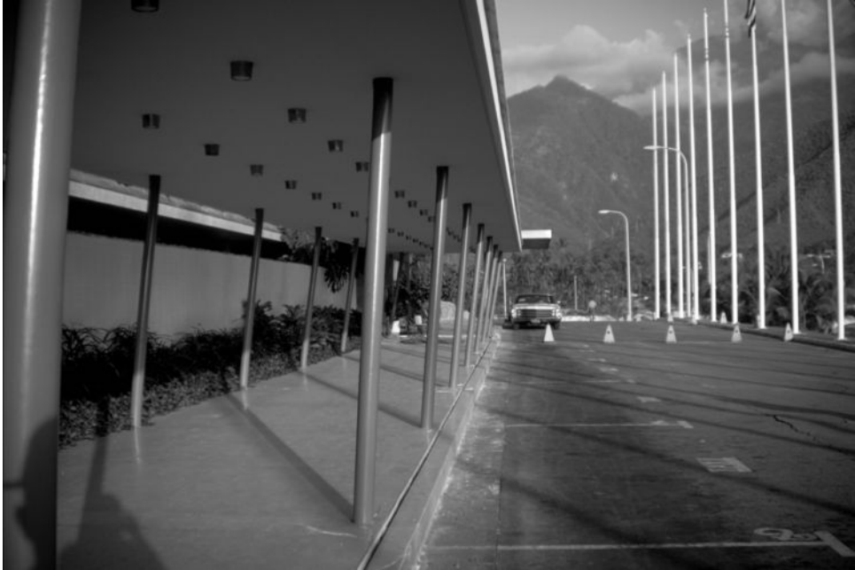
Figure 1.1.1 This pergola at the Macuto-Sheraton Hotel near Caracas, Venezuela, was damaged by earthquake on July 29, 1967. The Magnitude 6.5 event, which was centered about 15 miles from the hotel, overstrained the steel pipe columns, resulting in a permanent roof displacement of 9 in. (From the Steinbrugge Collection, National Information Service for Earthquake Engineering, University of California, Berkeley.)
