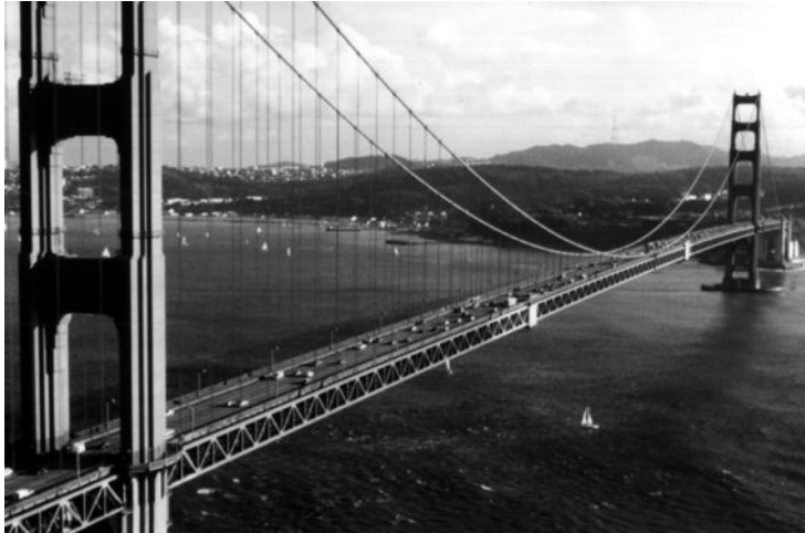
Figure 2.1.2e Golden Gate Bridge, San Francisco, California. The fundamental natural vibration periods of this suspension bridge with the main span of 4200 ft are 18.2 sec for transverse vibration, 10.9 sec for vertical vibration, 3.81 sec for longitudinal vibration, and 4.43 sec for torsional vibration. These vibration properties were determined from recorded motions of the bridge under ambient (wind, traffic, etc.) conditions. (Courtesy of International Structural Slides.)
