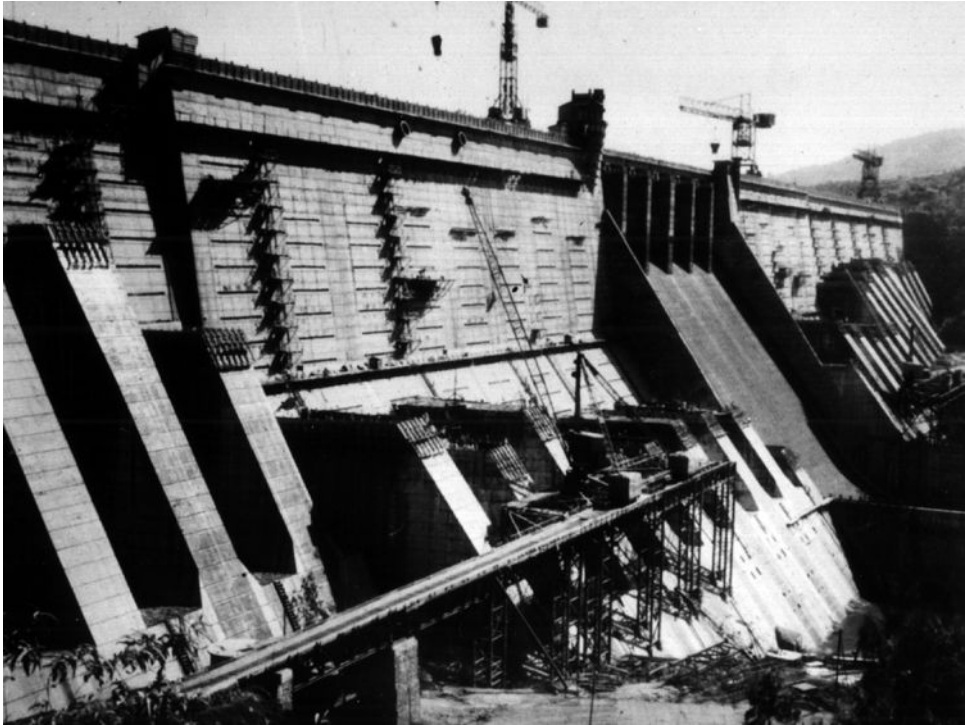
Figure 18.11.4 Addition of buttresses to Koyna Dam after the damage caused by the Koyna earthquake of December 11, 1967. [From A. K. Chopra, "Earthquake Response Analysis of Concrete Dams," in Advanced Dam Engineering for Design, Construction and Rehabilitation (ed. R. B. Jansen), Van Nostrand Reinhold, New York, 1988.]
