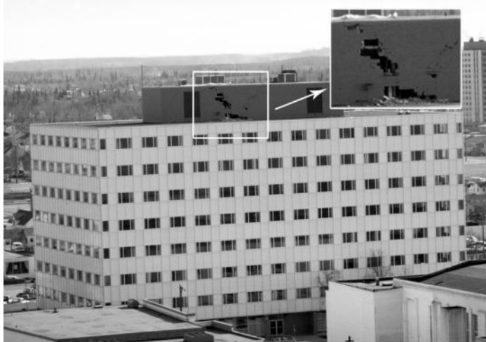
Figure 13.2.12 The Hill Building in Anchorage, Alaska, after the Prince William Sound earthquake, March 27, 1964, Magnitude 9.2. Except for the damage to the penthouse wall (close-up), the building was essentially undamaged. (From the Steinbrugge Collection, National Information Service for Earthquake Engineering, University of California, Berkeley.)
