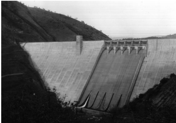
Figure 2.1.2d Pine Flat Dam on the Kings River, near Fresno, California. The fundamental natural vibration period of this 400-ft-high concrete gravity dam was measured by forced vibration tests to be 0.288 sec and 0.306 sec with the reservoir depth at 310 ft and 345 ft, respectively.
