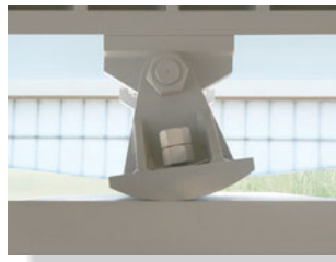
The rocker support for this bridge girder allows horizontal movement so the bridge is free to expand and contract due to a change in temperature. (4)
