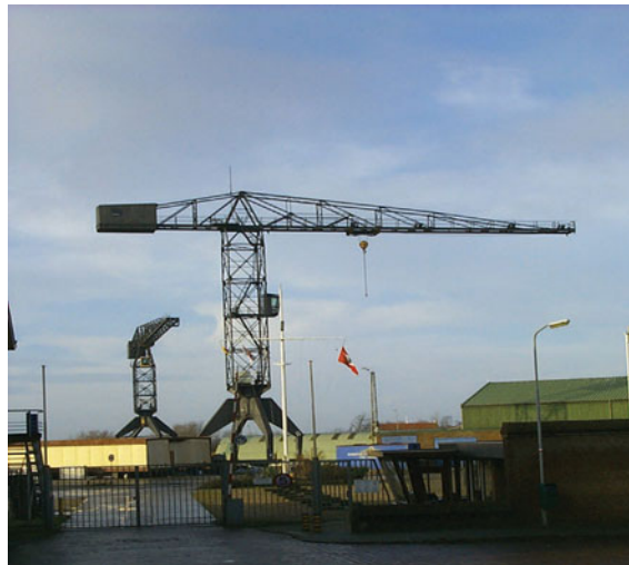
Simple trusses are often used in the construction of large cranes in order to reduce the weight of the boom and tower.
