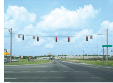
Each of the cable segments remains approximately straight as they support the weight of these traffic lights.
