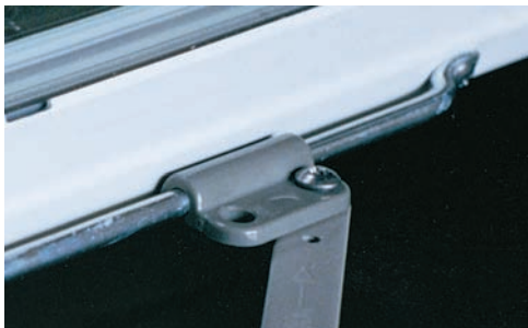
Photo 4.3 As the link of the awning window opening mechanism is extended, the force it exerts on the slider results in a normal force being applied to the rod, which causes the window to open.
