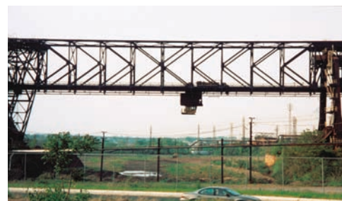
Photo 6.2 Two K-trusses were used as the main components of the movable bridge shown which moved above a large stockpile of ore. The bucket below the trusses picked up ore and redeposited it until the ore was thoroughly mixed. The ore was then sent to the mill for processing into steel.
