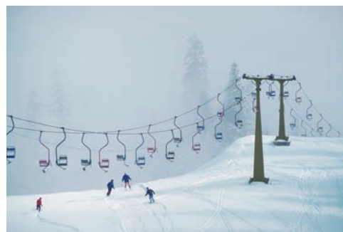
Photo 7.3 Since the weight of the cable of the chairlift shown is negligible compared to the weights of the chairs and skiers, the methods of this section can be used to determine the force at any point in the cable.
