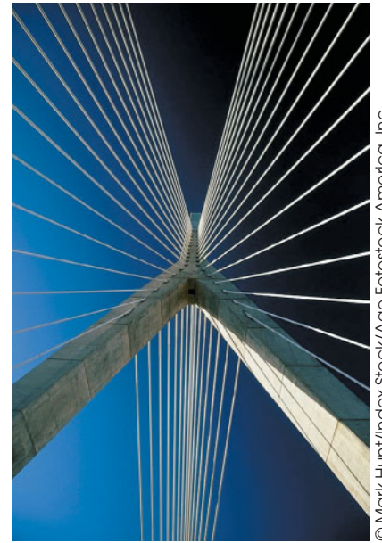
The three-dimensionality of the cable system on the Leonard P. Zakim Bunker Hill Bridge is evident in this view.
