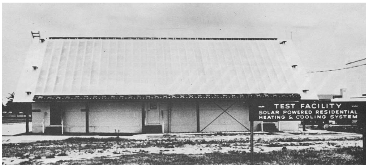
Fig. 17-14 This research solar-energy house is cooled by a lithium-bromide air conditioner. It uses solar-heated water. (Arkla)
