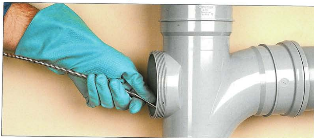
Use a hired auger to clear a soil stack
