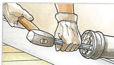
2 Use a cold chisel to cut out the remnants
