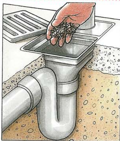
Bail out the water, then clear a gully by hand
