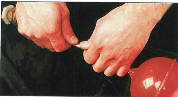
1 Straighten or bend a metal float arm
