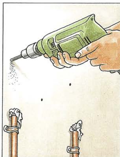
4 Drill and plug the holes
