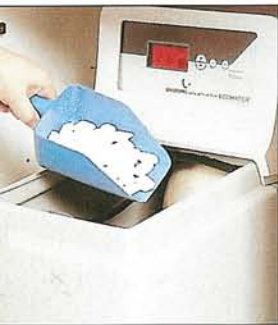
Water softener A domestic unit, which fits neatly beneath the worktop, requires topping up with salt.
