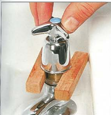
1 Jack the head off a tap with wooden packing
