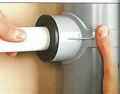
4 Push the waste pipe into the boss
