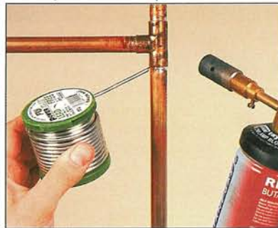
Introduce solder to a heated end-feed joint
