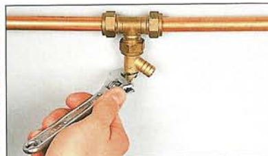
Tightening a leaking draincock
