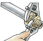
2 Tighten the coupling
