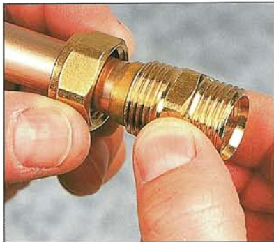
2 Clamp the joint to the pipe with the nut
