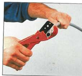
Cutting plastic pipe Polybutylene pipe is easy to cut, using special shears.
