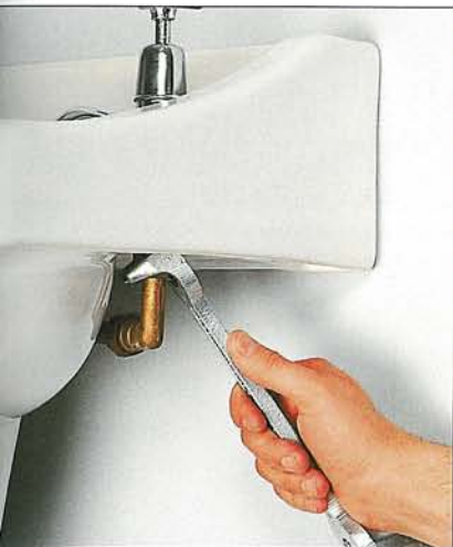
Releasing a tap connector Use a special cranked spanner to release the fixing nut of a tap connector.
