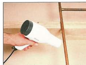
Thawing a frozen pipe Play a hairdryer gently along a frozen pipe, working away from the blocked tap or valve.
