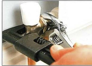
Grip leaky valve with wrench and tighten cap-nut
