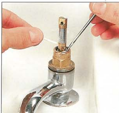
2 Stuff string or a thread of PTFE tape into the gland
