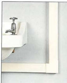
Hide your pipes inside plastic ducting
