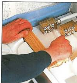
2 Push tubing into the distributors
