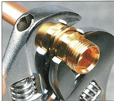
4 Tighten the joint with two spanners
