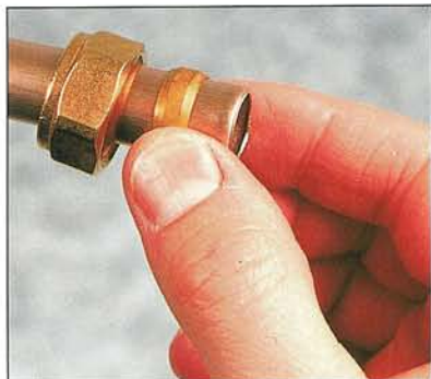
1 Slip an olive onto the pipe after the cap-nut
