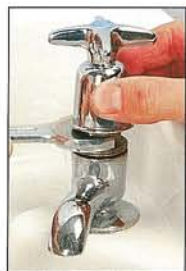
1 Loosen headgear nut
