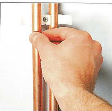
Clip pipes to the wall
