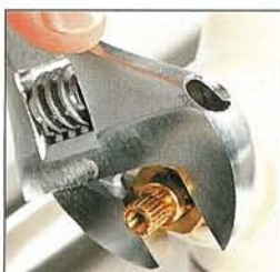
1 Unscrew the cartridge
