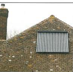
Mount collectors on a south-facing roof
