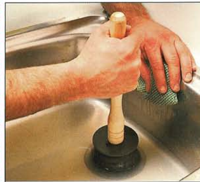
Use a plunger to force out a blockage
