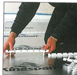
1 Press the pipe clips into place
