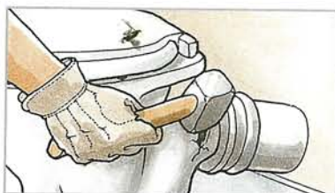
1 Break the outlet of the pan with a hammer
