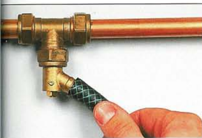
Attach hosepipe to draincock
