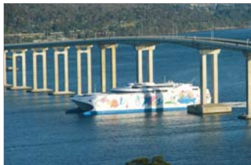
Figure 7. Hull 64, Nachan Rera, clears Tasman Bridge, Hobart, bound for open sea.
