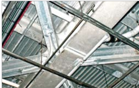
Figure 10. Separately mounted superstructure visible above sturdy sea frame cross bracing.
