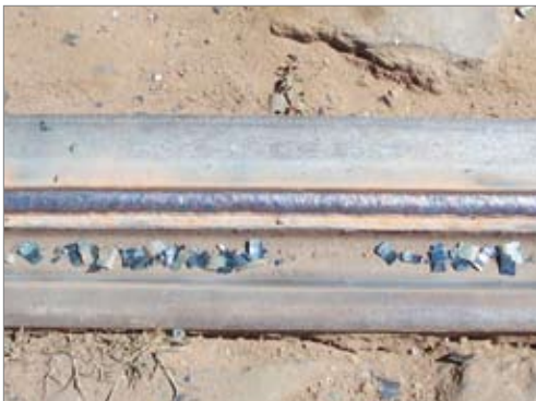
Figure 3. Deposited weld before and after slag removal.
