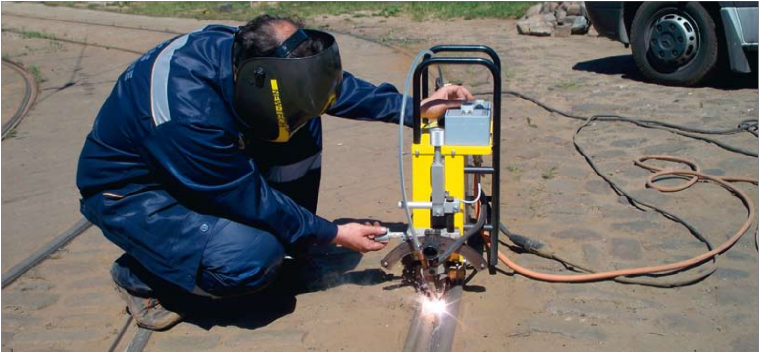
Figure 2. The curved slide on which the welding head is located enables easy and exact positioning of the wire extension.
