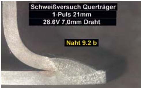
Figure 2. Weld penetration of an overlap joint in a cross support beam. t=2\text{mm} . 225A/130cm/min.min.
