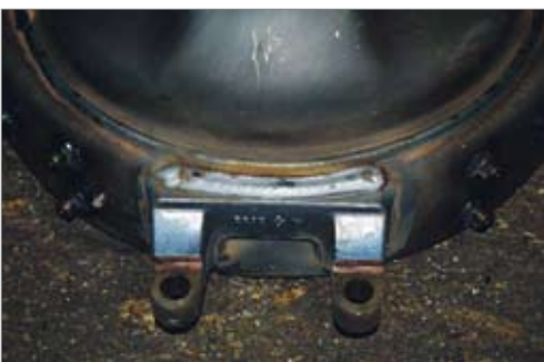
Figure 7. Good appearance of all welds.
