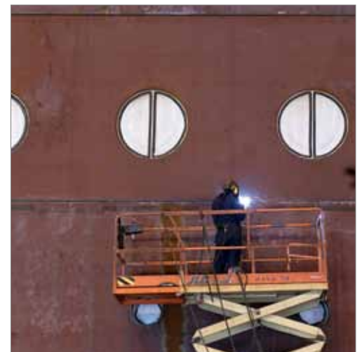
MAG welding with flux-cored wire.
