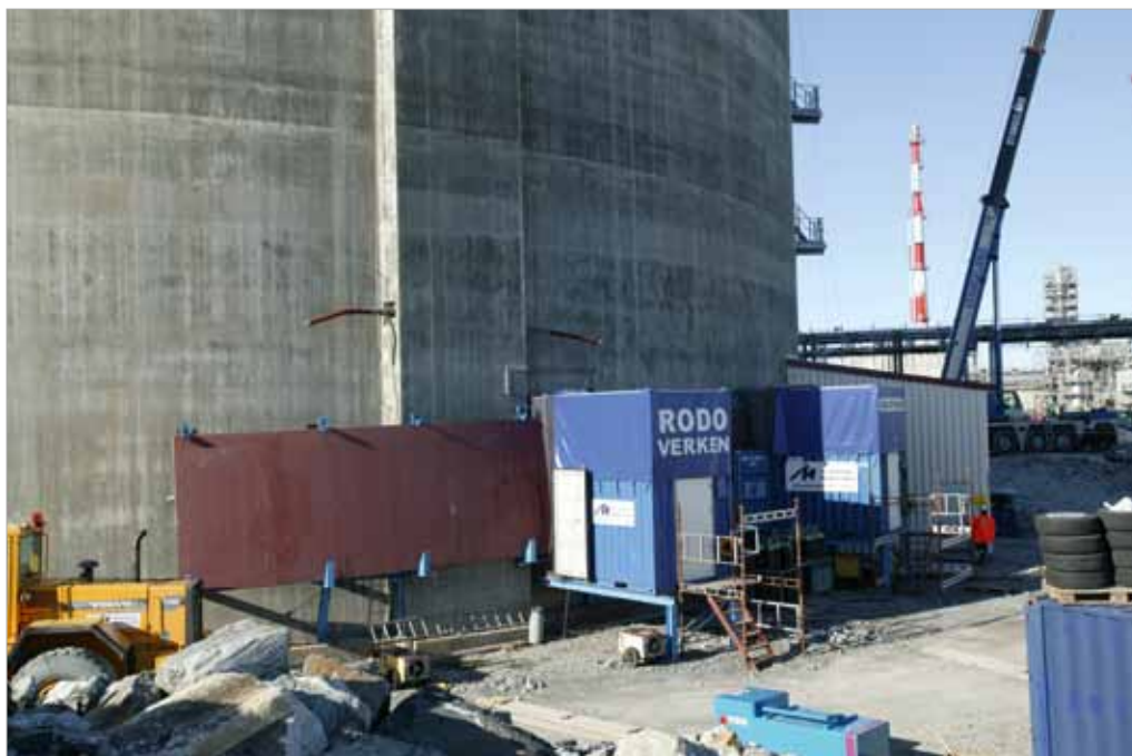
Figure 6. Joining of plates in PF position before they are fed into the tank's concrete outer wall. Welding process: mechanised MIG.
