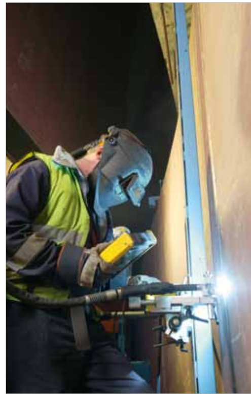
Figure 7. Welding of the first side of the vertical welds, taking place outside the concrete wall in a welding cabin.
