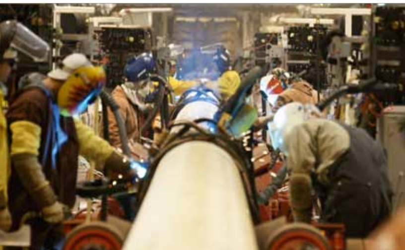
Figure 2. Firing line onboard Allseas' Audacia lay barge.
