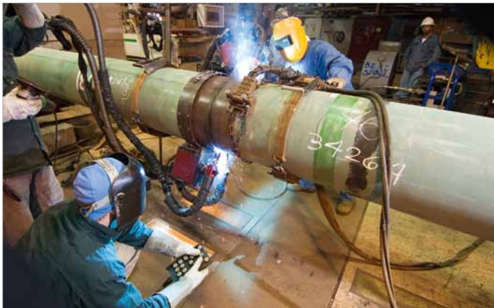
Figure 7. Welding of the root pass on the firing line with two single GMAW torches.
