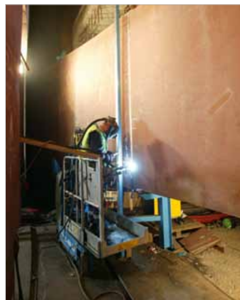
Figure 8. MIG welding of the reverse side of the vertical joint, in the work opening inside the concrete tank wall, using OK Autrod 19.82, AristoMig 500 power sources and Railtrac equipment for mechanised welding.
