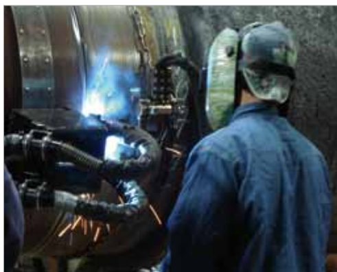
Figure 8. Welding of filler layers with two tandem SMAW torches.
